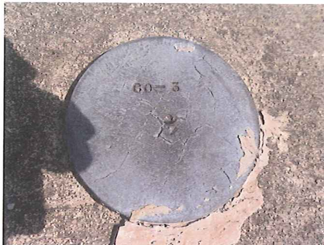
Photo - Station Detail
