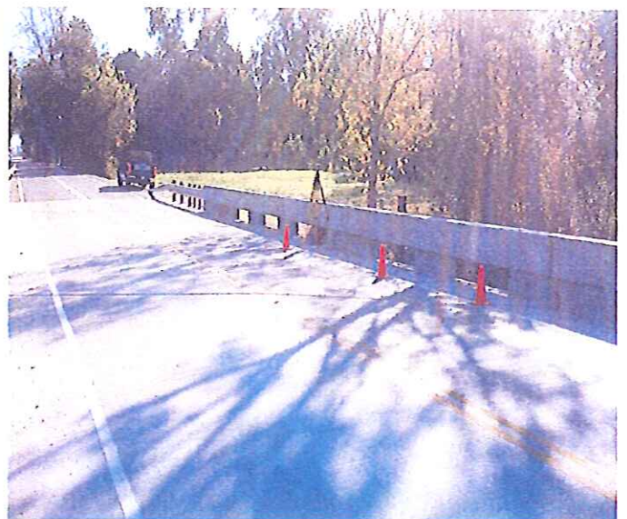
Photo - Station Area
